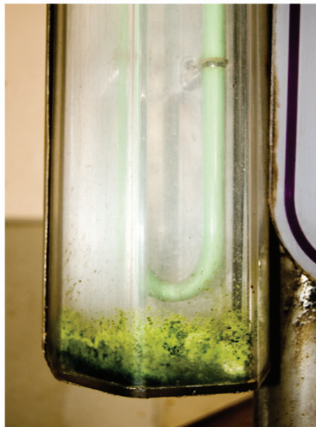
EXAMPLE 2. THIS SIGN WAS NOT CLEANED REGULARLY AND ALSO DID NOT HAVE PROPER DRAINAGE. AS A RESULT ALGY BUILT UP ON THE BOTTOM.
